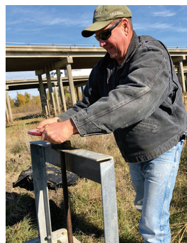
Farmer Mike DeWit (bottom left) adjusts the screwgate that maintains desired outflow and facilitates passage of the salmon out of the rice field. Crews deploy protective cages (bottom, right) to house juvenile salmon that will receive special telemetry tags enabling researchers to track their progress towards the Pacific Ocean (top).
